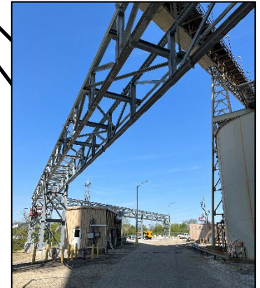
Flue Gas Ducting Bridge
