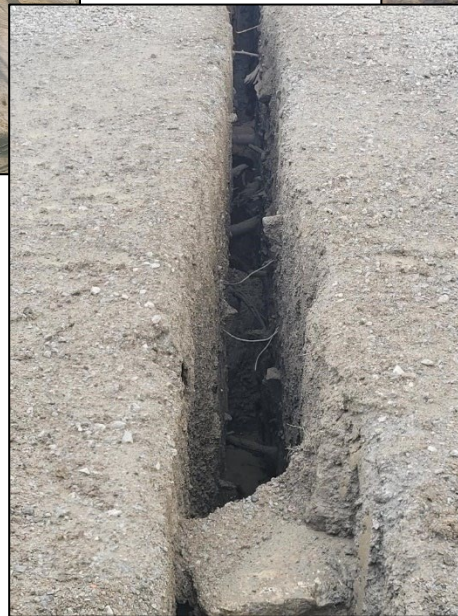
Hydroexcavation section revealing underground lines
