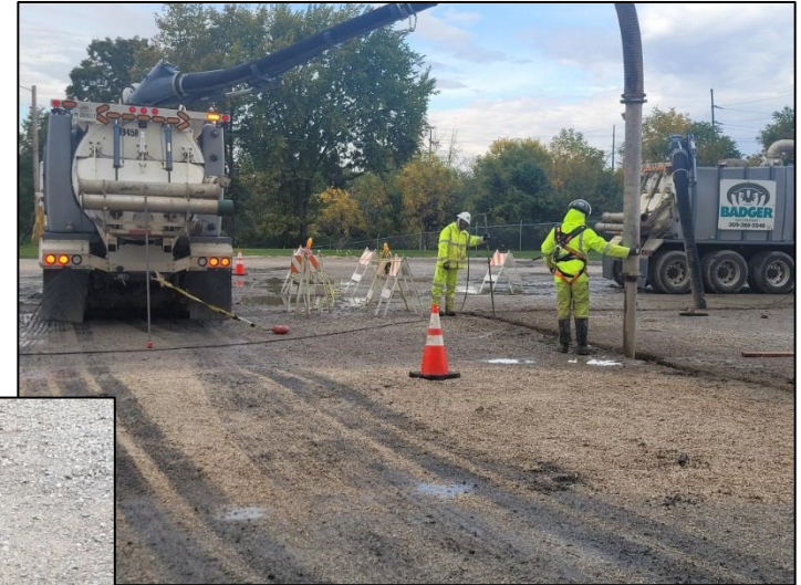
Hydroexcavation in action
