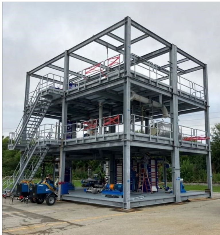
Off-site module fabrication
