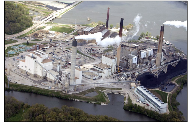
City Water, Light and Power (CWLP) in Springfield, IL
