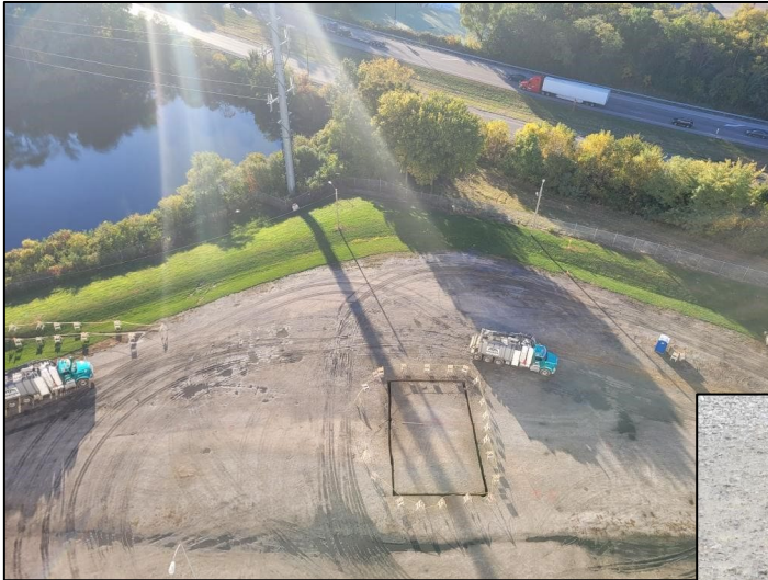
Completion of pit area perimeter hydroexcavation
