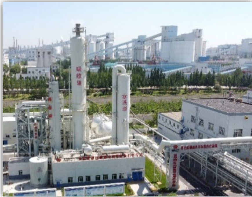
150,000 t CO 2 /y Power Plant Project China Energy Group, Yulin City, 2021
