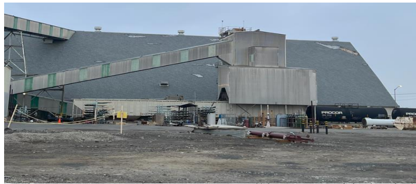
OCOchem Process Building
