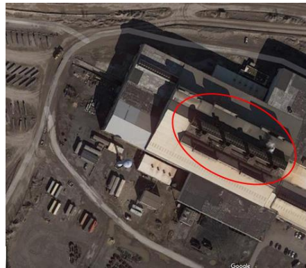
Tie-in to Waste Heat
