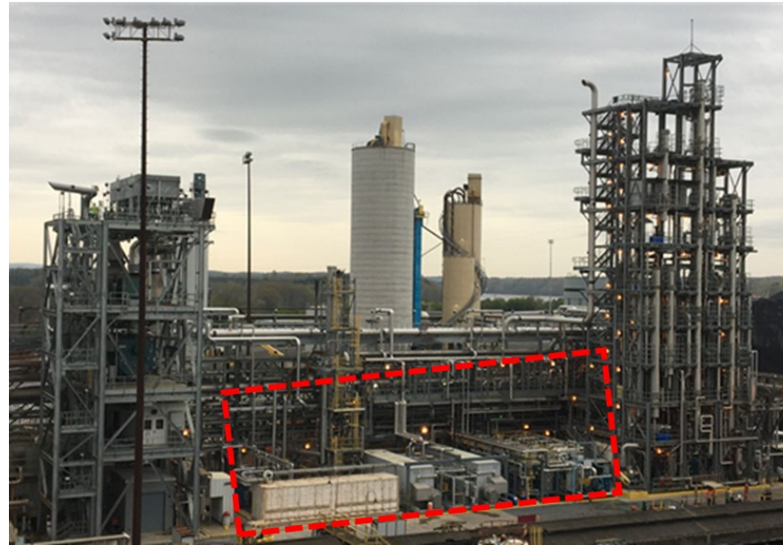
NCCC Pilot Bay Test Area
