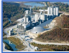
Holcim Ste. Genevieve Cement Plant Bloomsdale, Missouri
