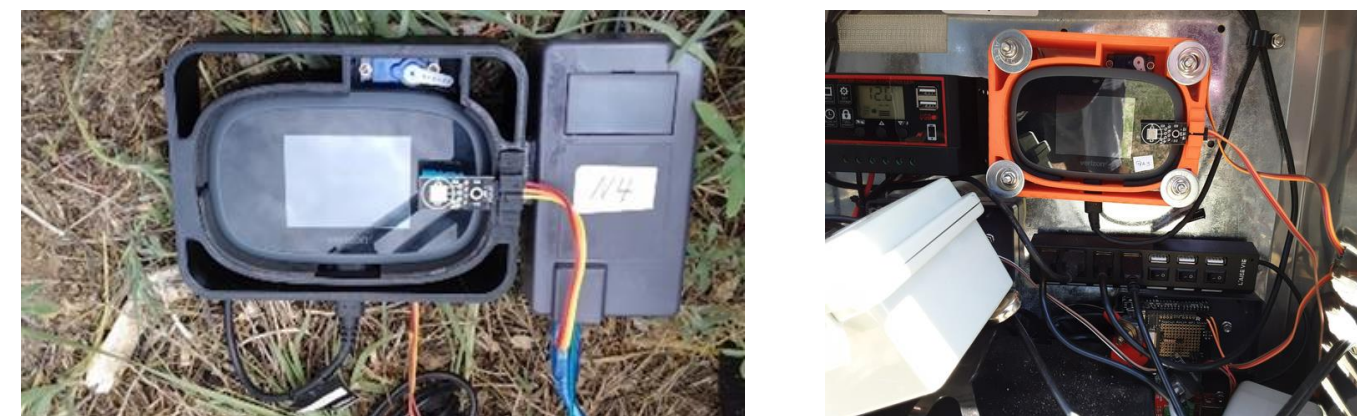
Figure 19-20. Deploying robot in field (left). Placing robot in new enclosure (right).
