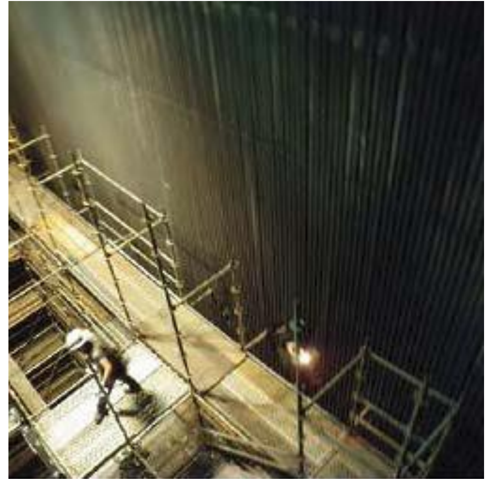
Hayden Unit 1 scaffolding for manual inspection and repair
