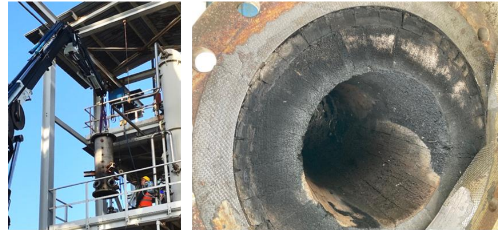
Reactor removal and refractory layer before the reconstruction
