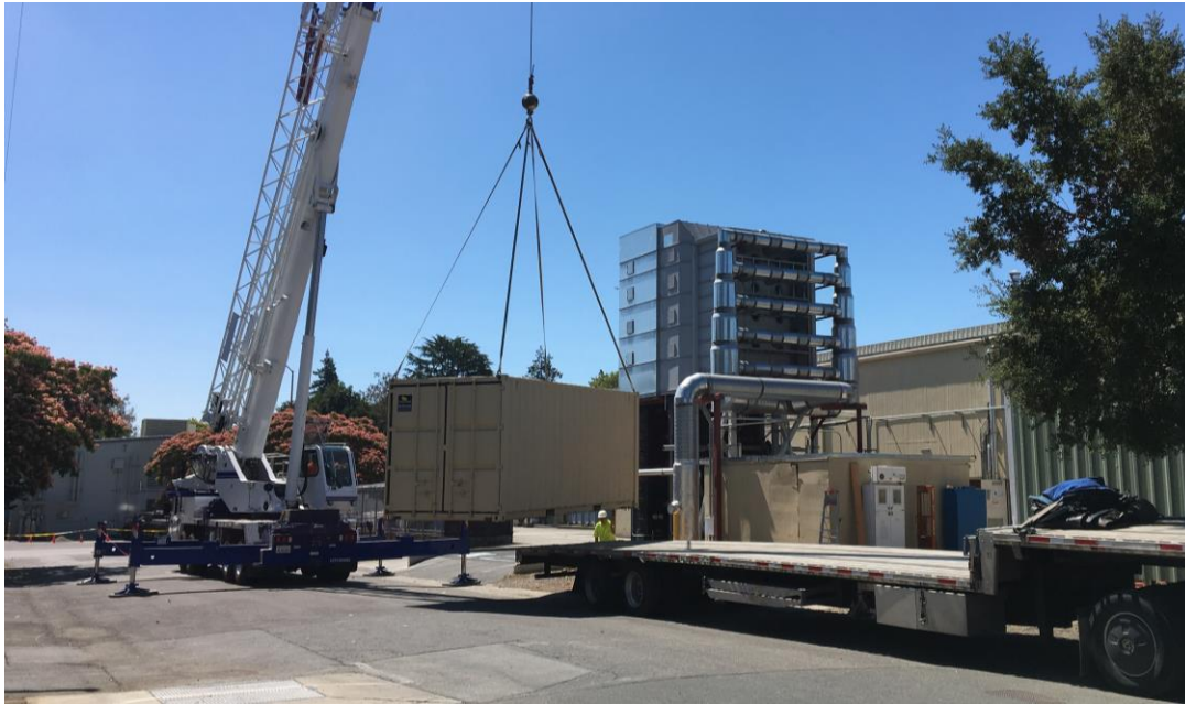
Skid Container being lifted onto trailer
