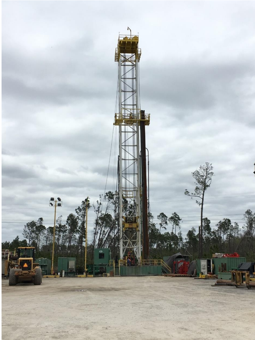
Electric rig drilling injection well TIW-2
