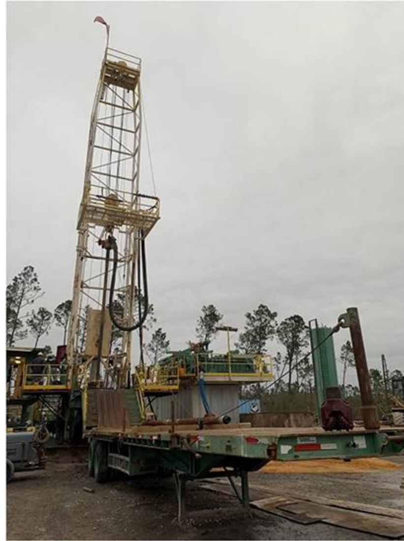
Diesel rig drilling extraction/observation well TEMW-A
