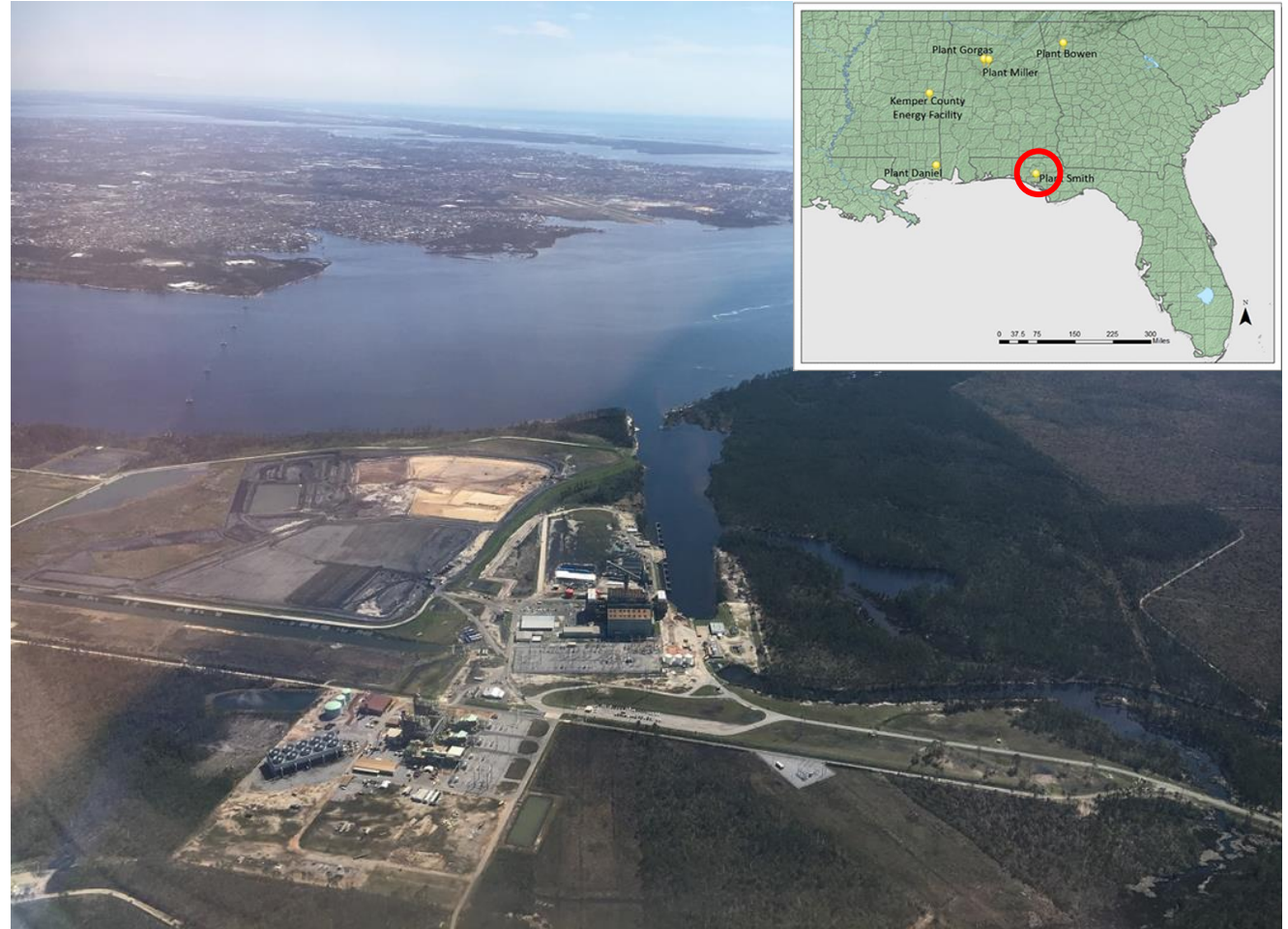
Photo showing Plant Smith in foreground and Panama City in background. Inset shows the location of Plant Smith in the Florida Panhandle (red circle).
