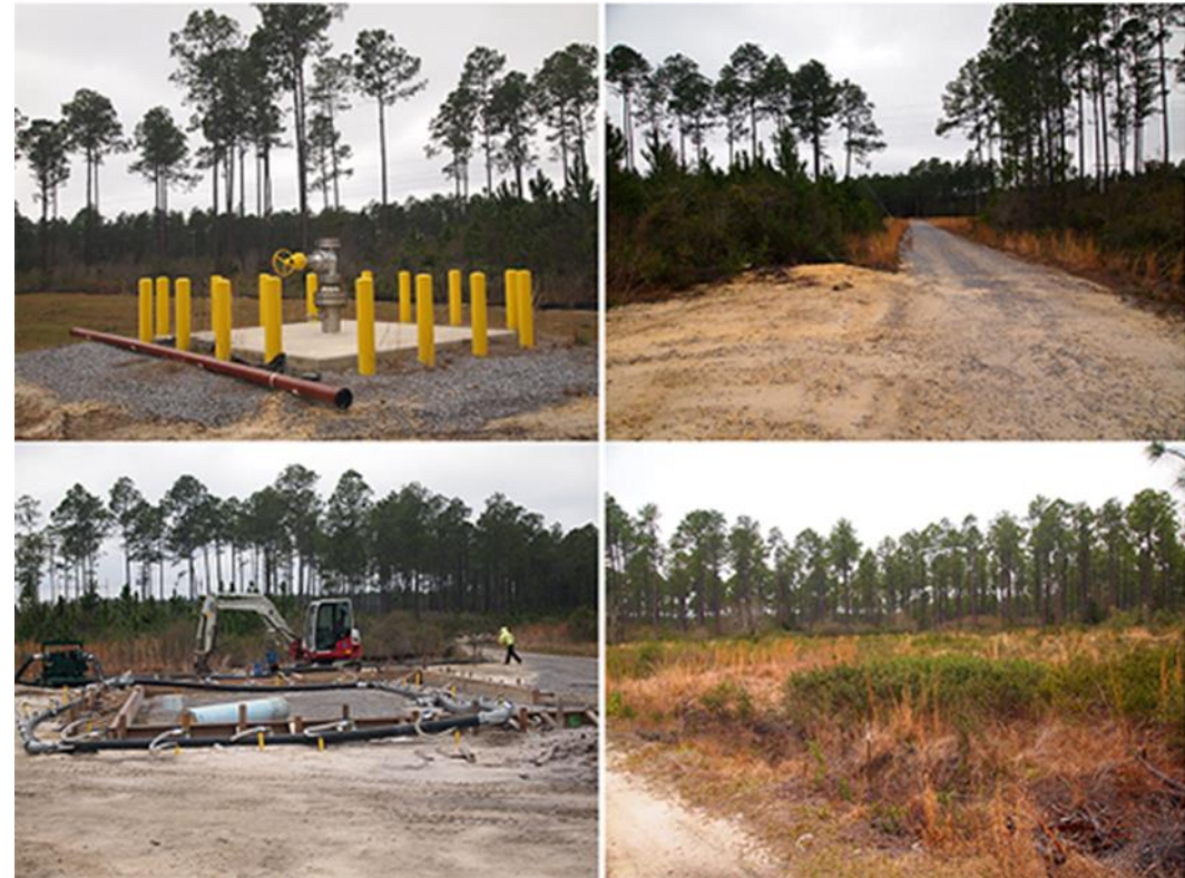
Photographs of existing Gulf Power wellfield. Photos clockwise from upper left: Eocene Injection well EIW-4; graveled access road; pump station under construction; cleared and permitted drilling pad location for future well
