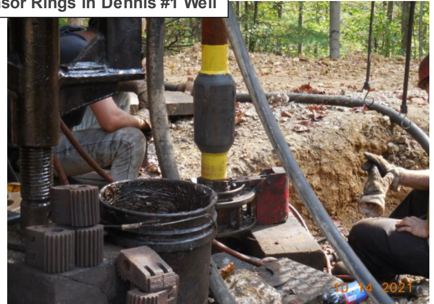
Running 4 ½" casing with Sensor Rings in Dennis #1 Well
