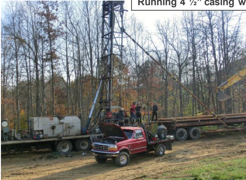
Running 4 ½" casing with Sensor Rings Hickenbottom #1 Well
