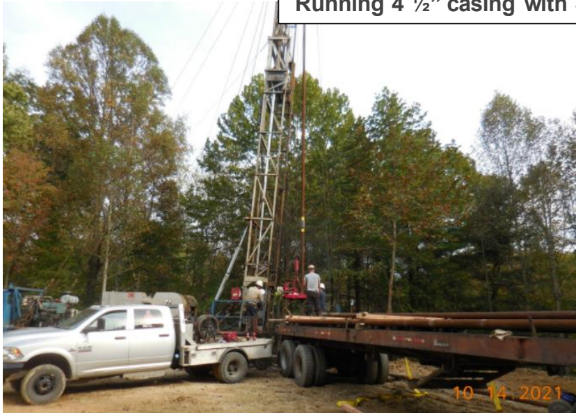
Running 4 ½" casing with Sensor Rings in Dennis #1 Well
