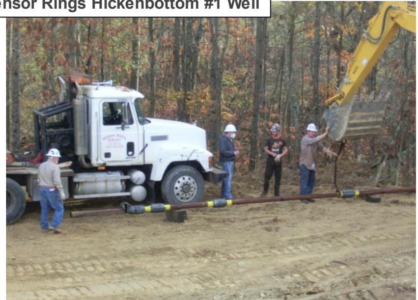
Running 4 ½" casing with Sensor Rings Hickenbottom #1 Well
