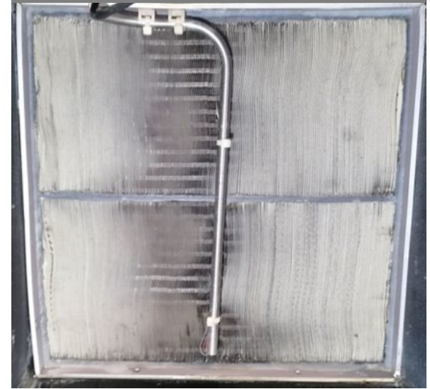
Steam outlet / air inlet, after 4546 cycles
