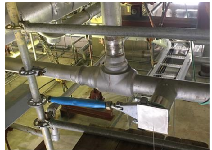
Tee welded in place at plant site, Net Power
