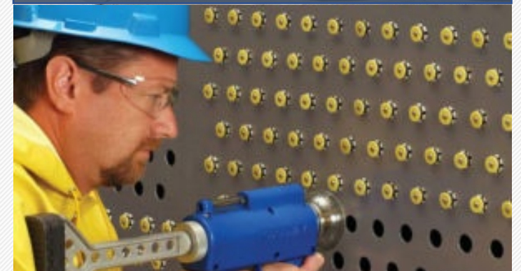
Mechanical Cleaning of Condenser
