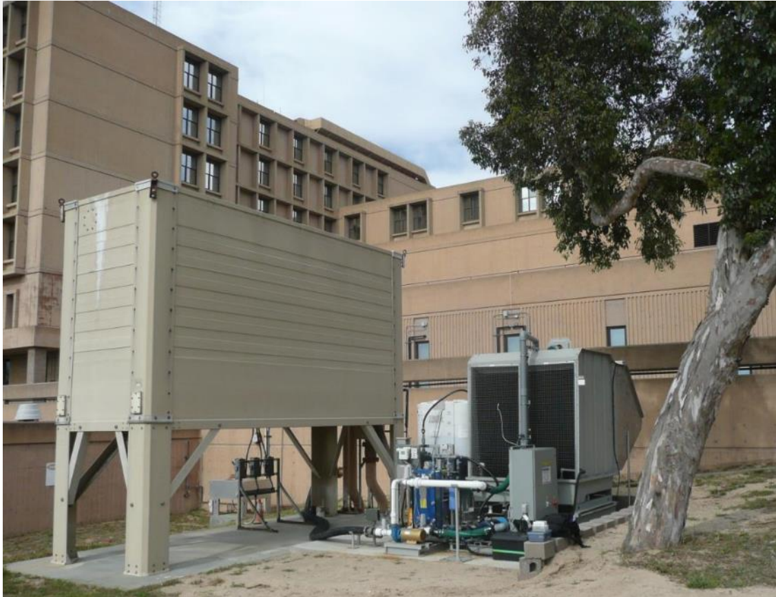
Field testing of a hygroscopic cooling tower in 2019.
