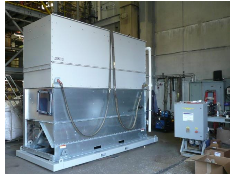
Hygroscopic cooling tower modifications underway at the EERC.
