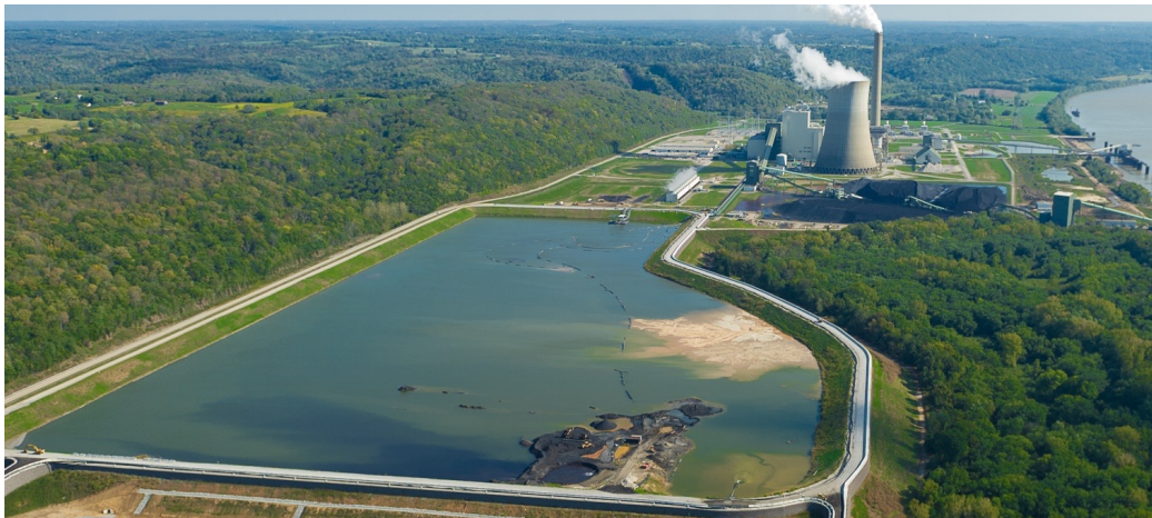
Trimble County Generating Station
