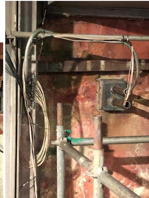
Penthouse Casing Penetration
