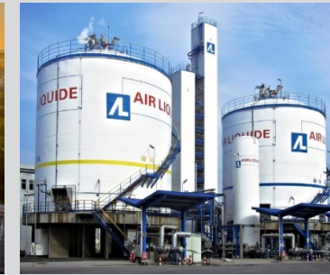
Air Liquide Liquid O 2 Storage
