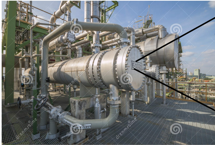
Heat exchangers in power plant
