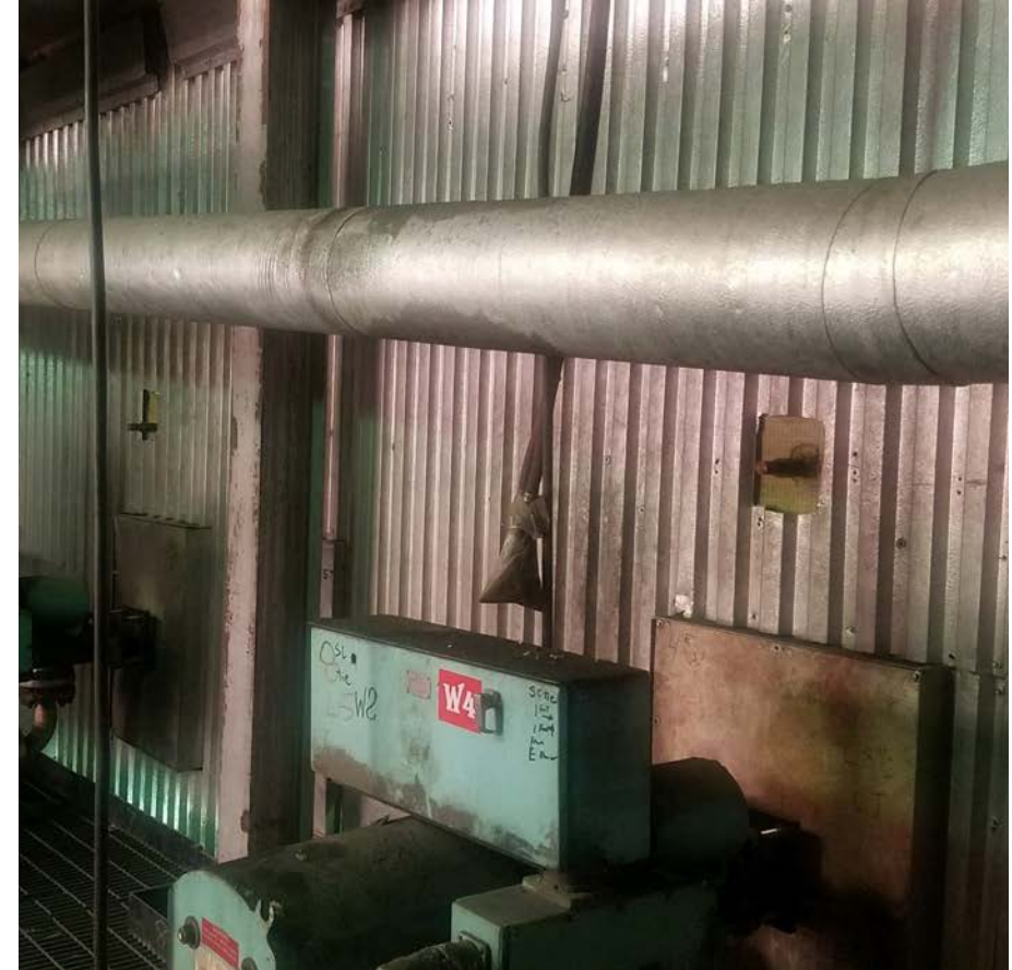
A wider view shows two of five installed waveguides
