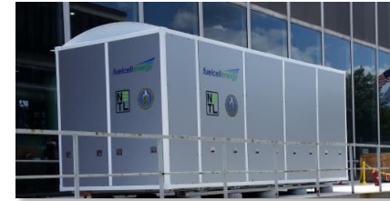
200kW Power Generation System Sub-MW / SOFC-GT Hybrid
