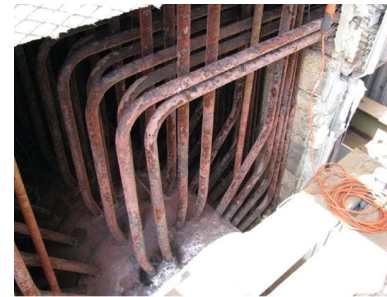
Reheater outlet header and tube-to-header weld fatigue damage as a result of thermal loading and deflection during startup cycles.
