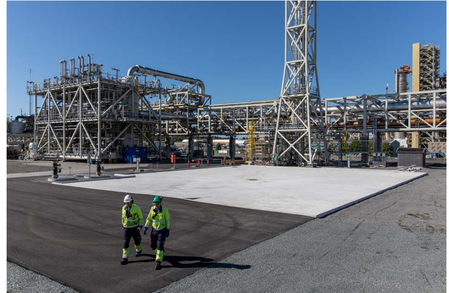
Close up view of 3 rd site foundation
