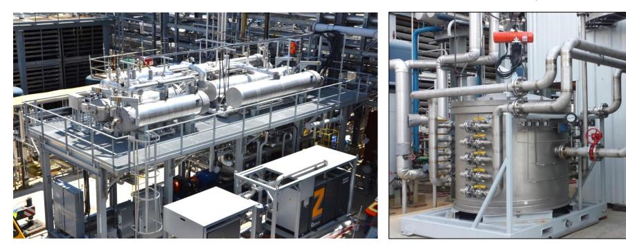
Spiral modules had large feed-to-residue pressure-drops and a large footprint
