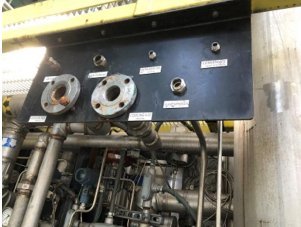
All Inter-connects have been disassembled
