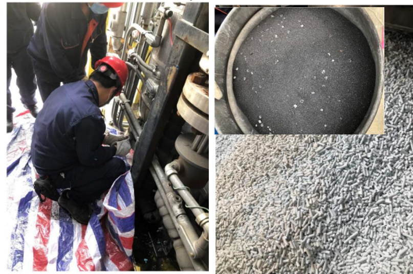
Sorbent and Catalyst have been unloaded
