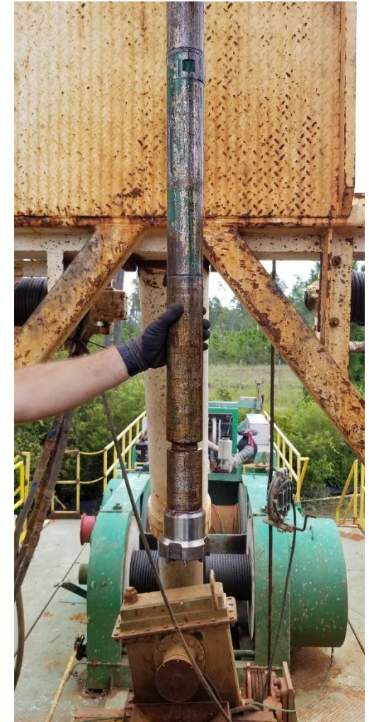
Mudmotor used to clear debris from the casing
