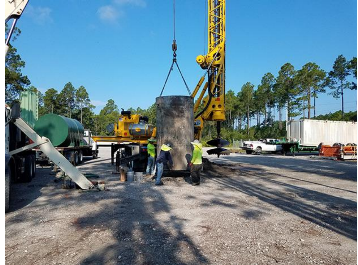
Installation of the 48-inch conductor casing
