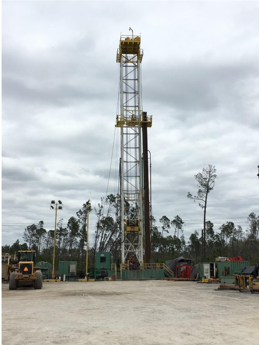
Electric rig drilling injection well TIW-2
