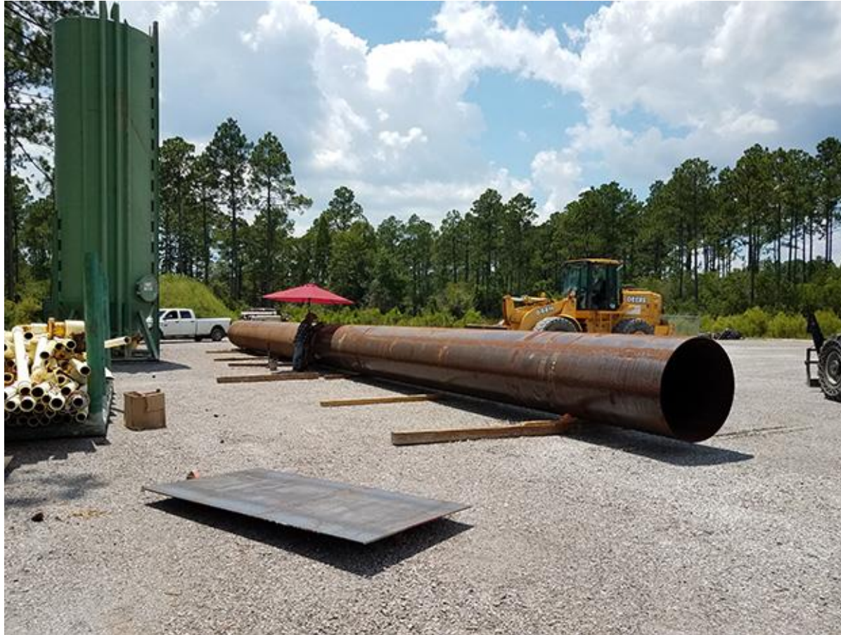
Welding sections of 48-inch dia. conductor casing together
