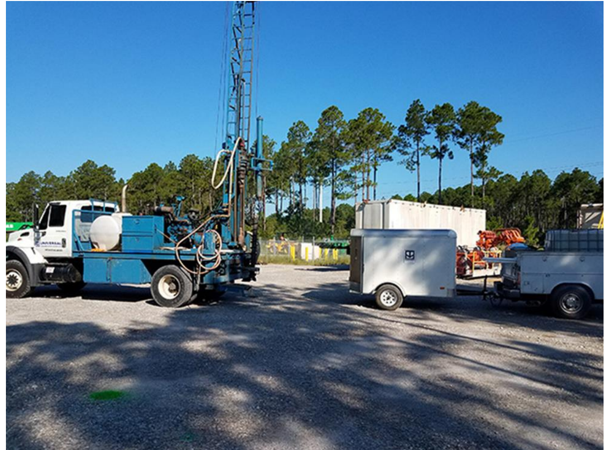
Monitoring well installation
