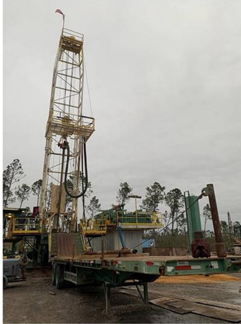
Diesel rig drilling extraction/observation well TEMW-A
