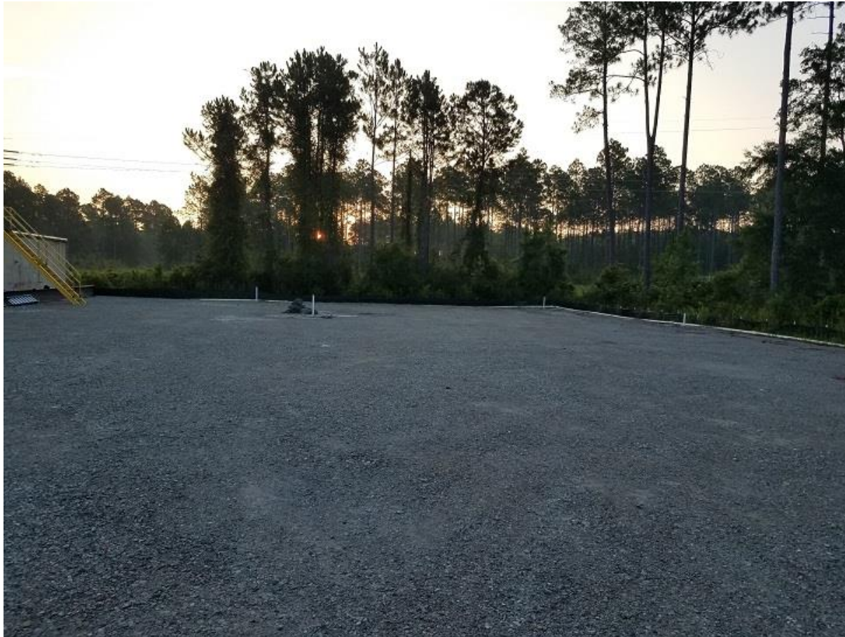
Drill pad installation
