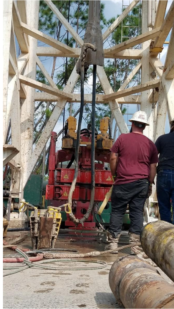
Fishing operations with tremie pipe looped back on itself
