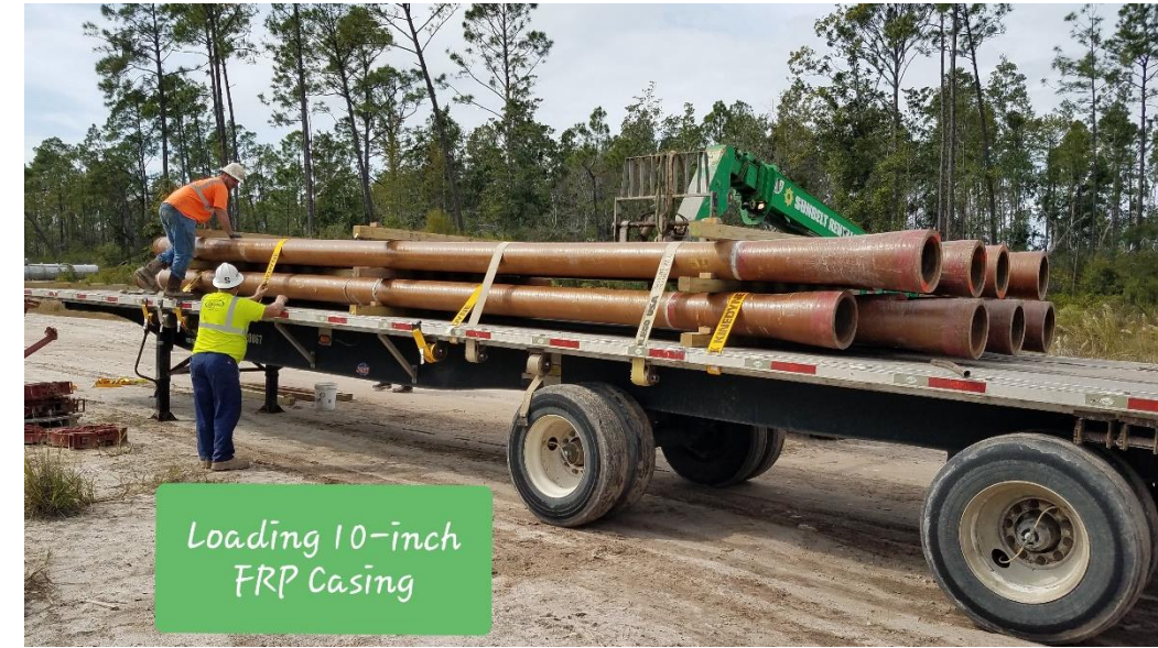
Free FRP casing was removed and shipped to manufacturer (bottom) and the rest was milled out (top)
