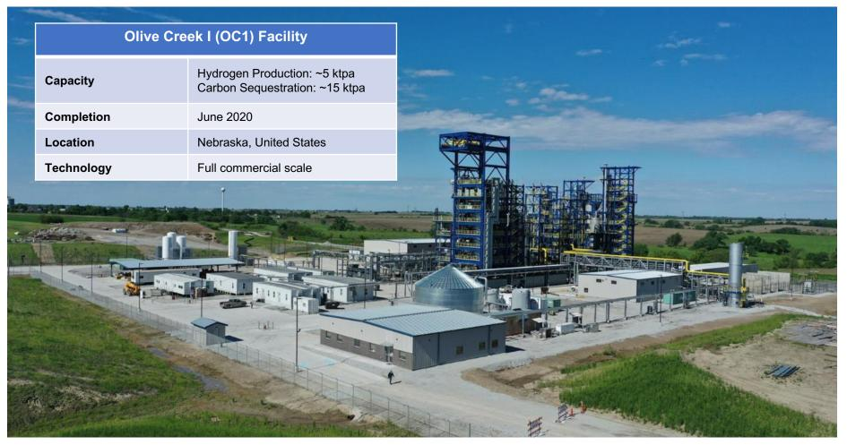
OC1 is the first commercial-scale methane pyrolysis facility built in the U.S.
