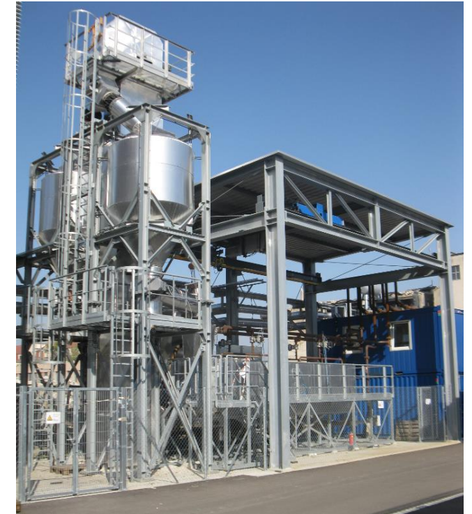
280-kWth pilot plant
