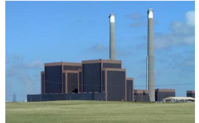
Coal Creek Station host site.
