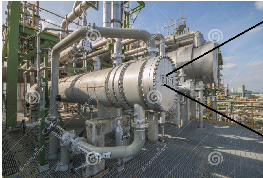
Heat exchangers in power plant
