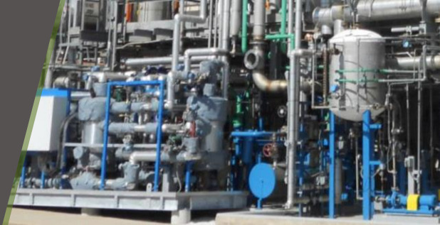
Pilot absorber/stripper system with high temperature flash skid
