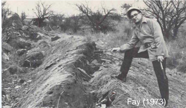
Fay (1973) Surface fracture, Elk City Blowout (Natural Gas Storage)
