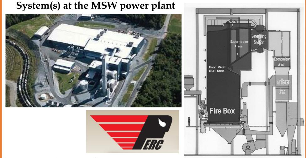
Power plant conditions: ✓ Temps ↑ 900°C (1650°F) ✓ Highly erosive/corrosive exhaust gases
