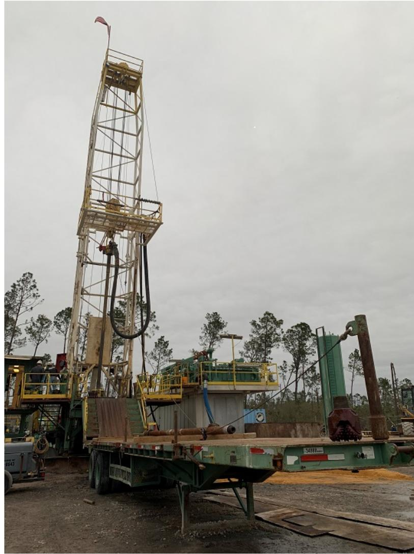
Diesel rig drilling observation well TEMW-A
