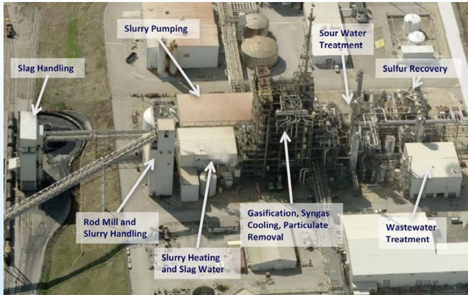
Aerial view of the WVR facility with various components of the syngas to ammonia process.
