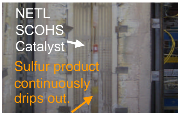
Sulfur removal using SCOHS catalyst
