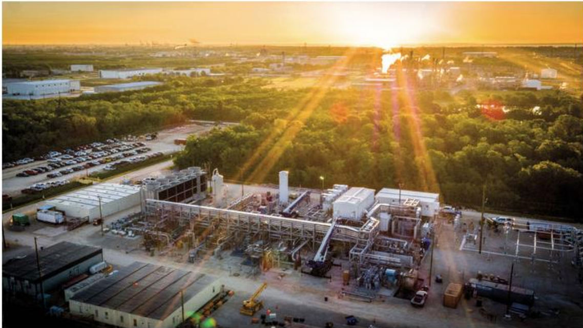
The prototype NET Power plant near Houston, Texas, is testing an emission-free technology designed to compete with conventional fossil power.
