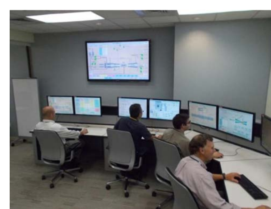
Monitoring of energy conversion systems.
