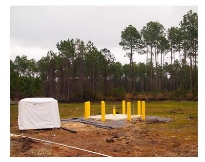
Permanent monitor well installed within 150 ft of injection well is sampled quarterly for water quality impacts associated with injection
