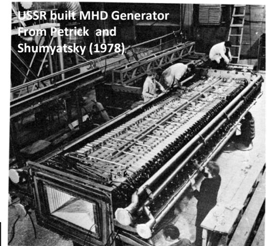
*MHD generator concept proven in 1980s w/ grid transferred power in both U.S. and USSR*
