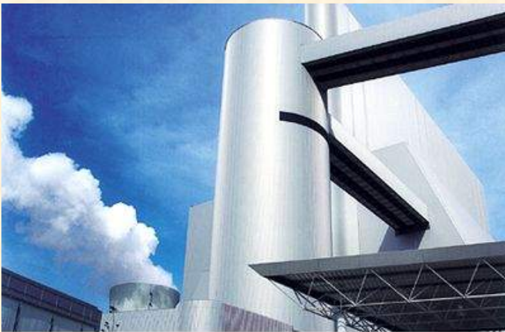
2 x 800 MW Lignite-Fired Power Plant Schwarze Pumpe, Germany
