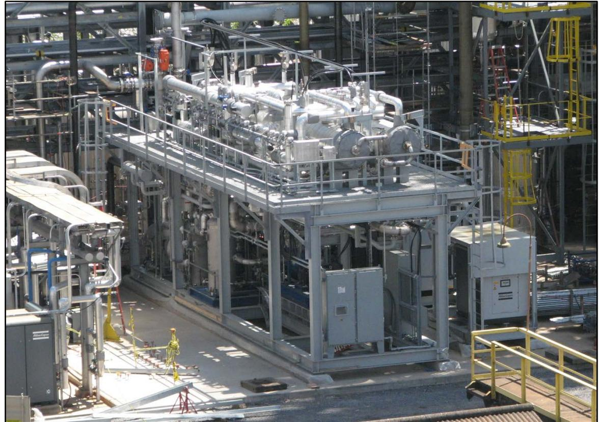
Data collected and lessons learned on MTR's 500 lb/hr flue gas bench-scale membrane used to support design and equipment selections of 10,000 lb/hr pilot-scale membrane.
