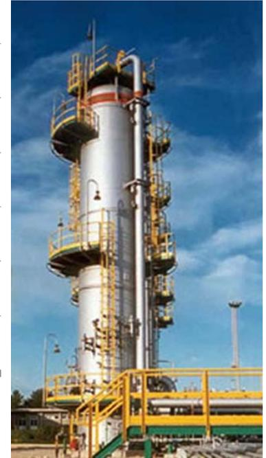
Enhancement over 10X reduces the absorber height to less than 130 feet for a 550 mWe coal-fired power plant\*
