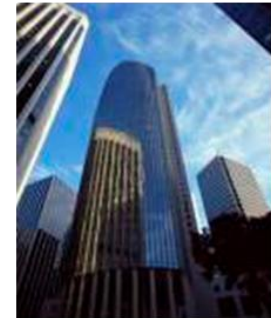
Commercial Power Stationary Power Units
