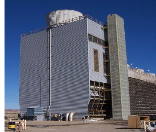
Air2Air™ condensing technology San Juan Generating Station
