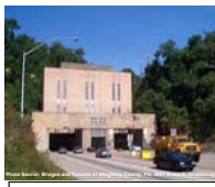
The western portal of the Squirrel Hill Tunnel
