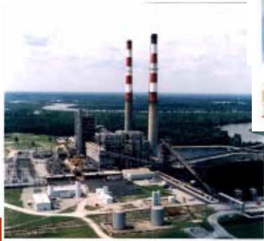
L.V. Sutton electric generating station
