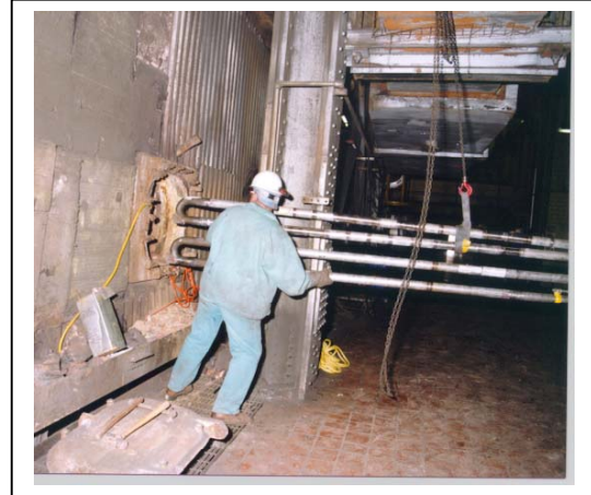
Figure 7: Installation into Niles Boiler
