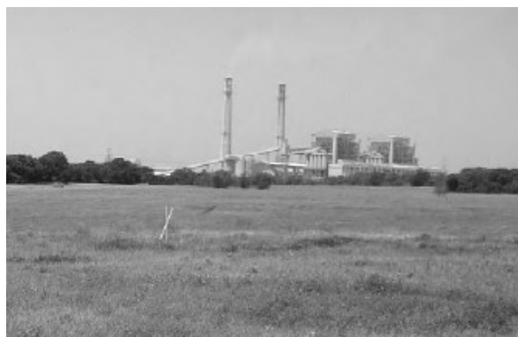
Proposed Jewett Power Plant Site (NRG Limestone Generating Station in the background)
